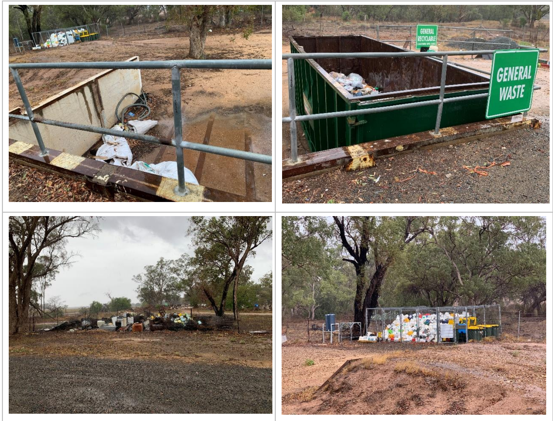
Photo 4.3 Tomingley WMF site photos
